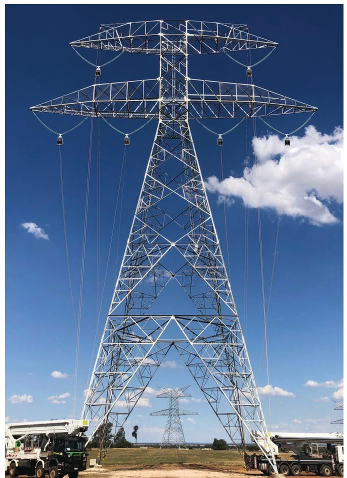
Danubio tower at Lockhart, NSW.
