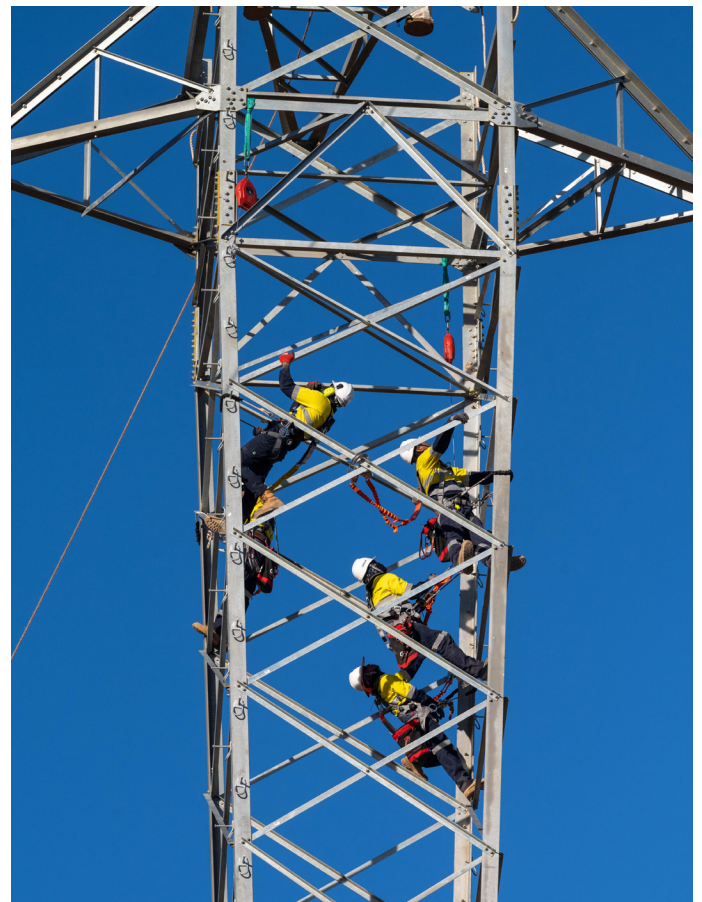
Riggers work at a tower at Buronga.
